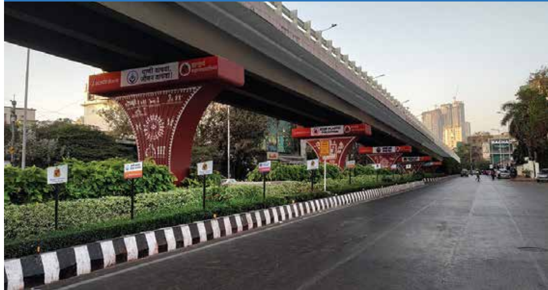
Worli Bridge – Love Groove
